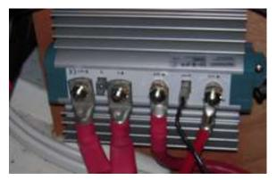
On this page are samples of equipment and their very neat installation. All wiring observed is properly routed and harnessed. Terminals are well protected at the AC level and DC terminals at the batteries are well protected and secure.
